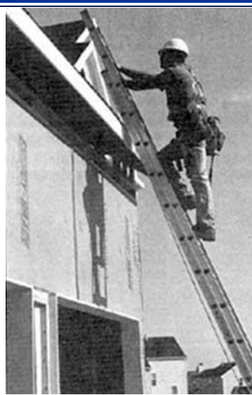
Figure 10. This worker is climbing a ladder set at the proper angle (4:1) with a three-point contact grip (two hands and one foot).
