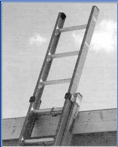
Figure 9. When ladders are used for access to an upper level they must extend at least 3 feet above the roof surface.
