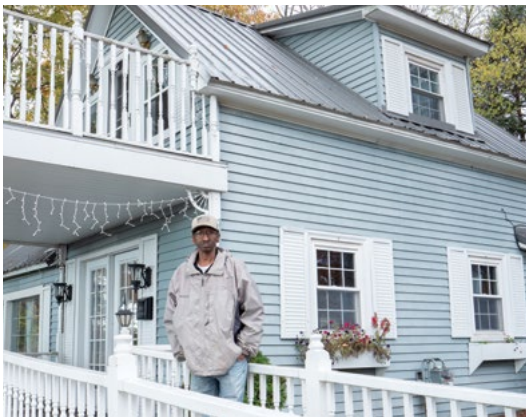
In 2020, we replaced a failing roof on veteran McCurdy Brown's home near Fife Lake.
