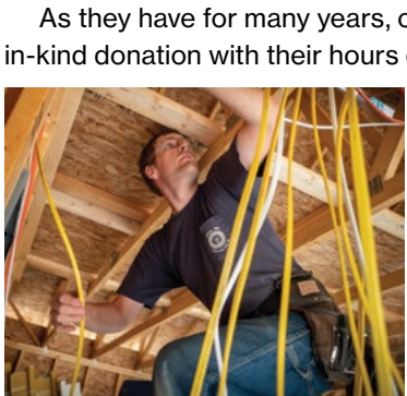
Professional electricians from the IBEW volunteered their skills and time in 2021.
